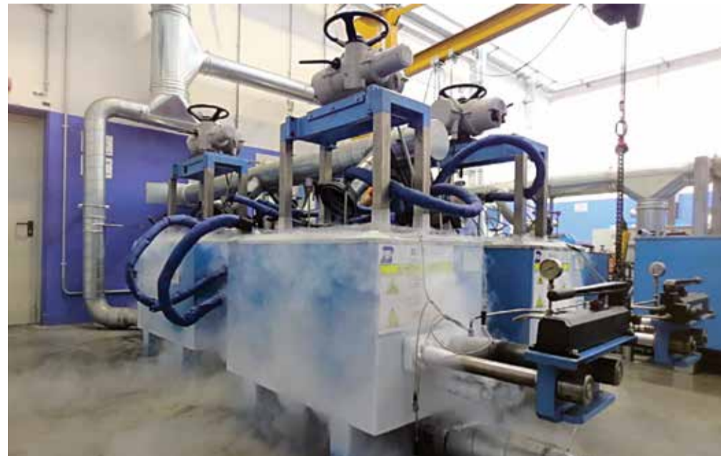
Bonney Forge Europe's in-house cryogenic test bunker allows for production testing of a wide variety of cryogenic valves for the LNG market.
